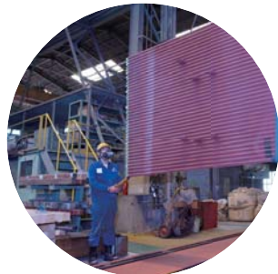
Thermal spraying onto boiler panels
