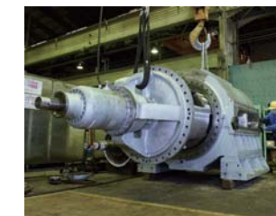
Feeder Overhaul of feeders
